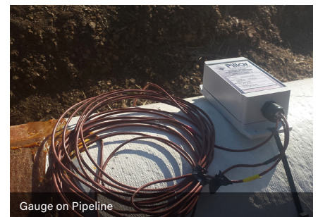
Gauge on Pipeline
