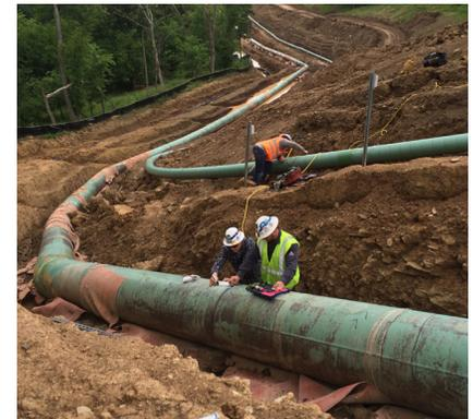
To gather data, the team partnered with a Professional Engineering firm specializing in pipeline stress analysis. This firm used available pipeline tallys and as-built drawings in order to recommend an excavation plan, recommend monitoring locations, and generate a stress profile of each pipeline using finite element analysis (FEA).
